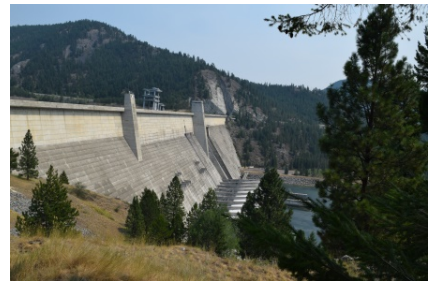
Libby Dam, Montana
